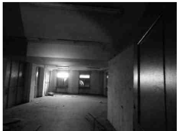
Current building - current floor 218 Calea Victoriei, District 1, Bucharest
