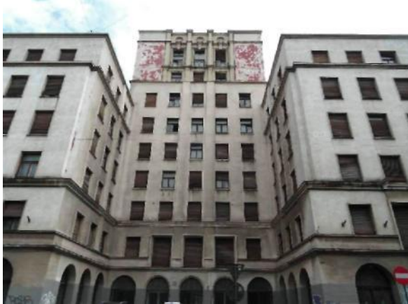
Current building - facade of Unit A 218 Calea Victoriei, District 1, Bucharest
