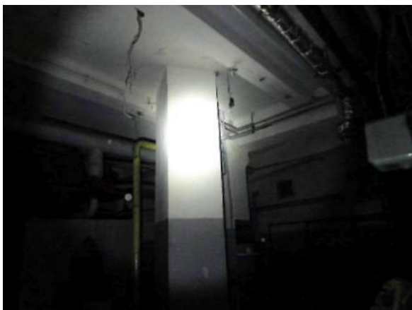
Current building - basement 218 Calea Victoriei, District 1, Bucharest
