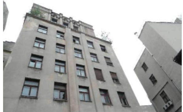
Current building - facade of Unit A 218 Calea Victoriei, District 1, Bucharest
